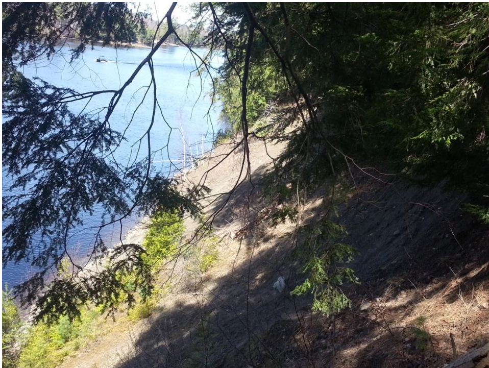
Photograph 2 – Illustrates the slip failures observed along the slope face near Slope Cross Section A.
